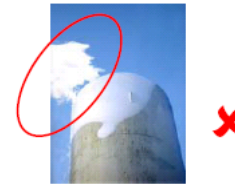
This picture shows gas venting from a vacuum protection device
