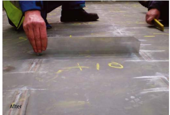
Distortions levelled after flame straightening
