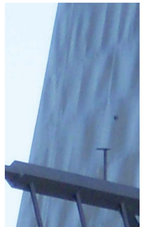
Visible distortion in a steel hull
